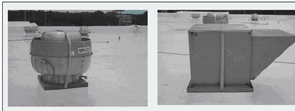
Heavy stainless steel straps attached to the curb with No. 14 screws.
